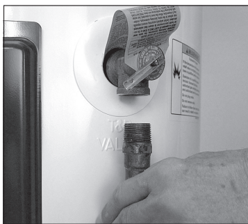
Removing the T&P Relief Valve discharge pipe.
