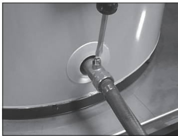
Draining the old water heater.
