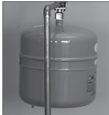
The Thermal Expansion Tank should be pressurized with air, to match the home's incoming water pressure.
